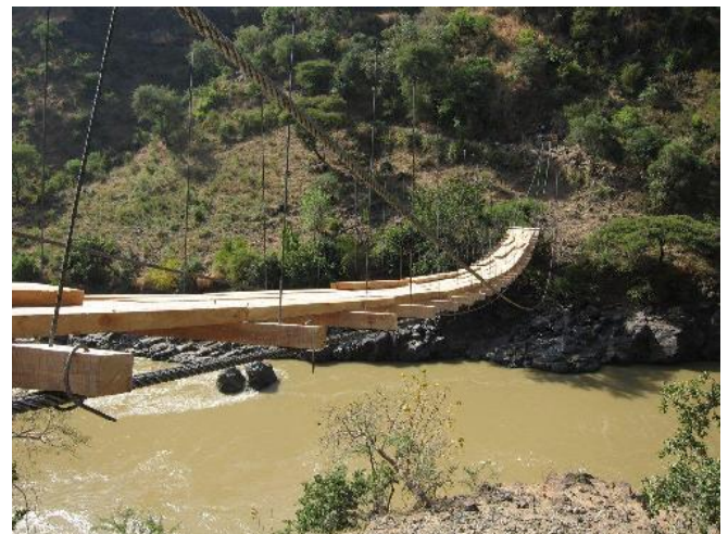
The bridge almost completed
